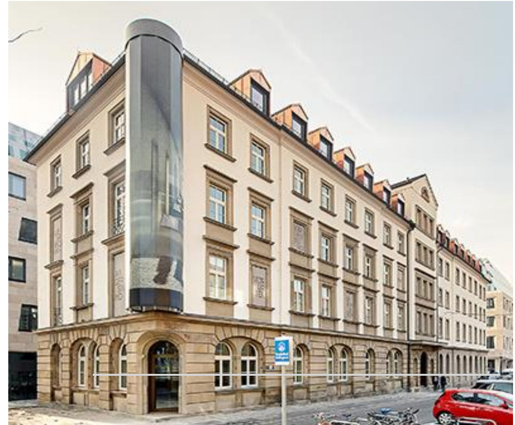
The Hotel Silber, former headquarters of the Political Police (Gestapo), is a location tied to Nazi perpetrators
